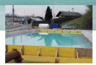
$\ensuremath{\text{CO}}_2$  storage reservoir of a construction site neutralisation plant
