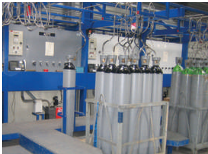
Filling station for high-purity gases
