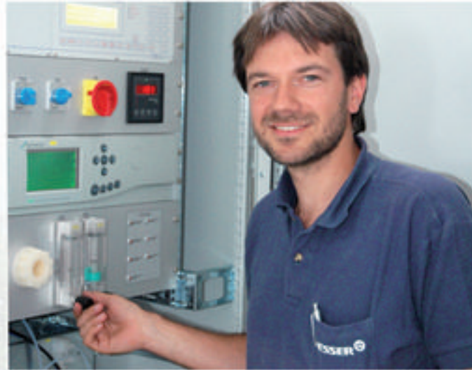
Disposal is fully automatic. Compliance with permissible emission levels is constantly monitored and documented.
