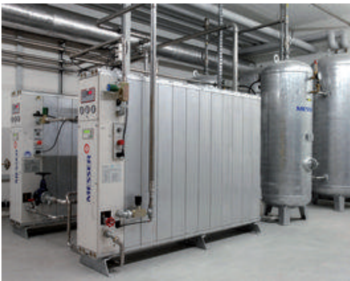
PSA unit for the production of nitrogen
