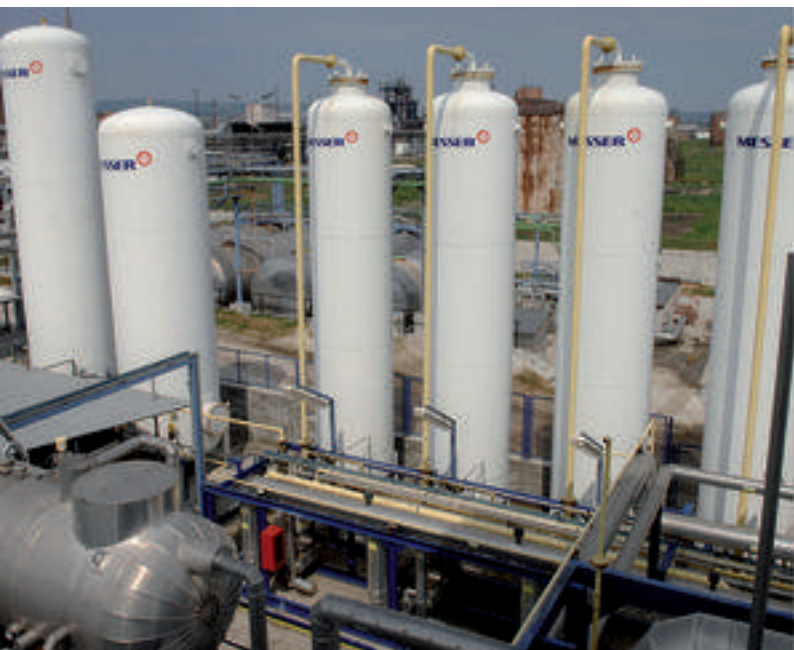
PSA unit for hydrogen production
