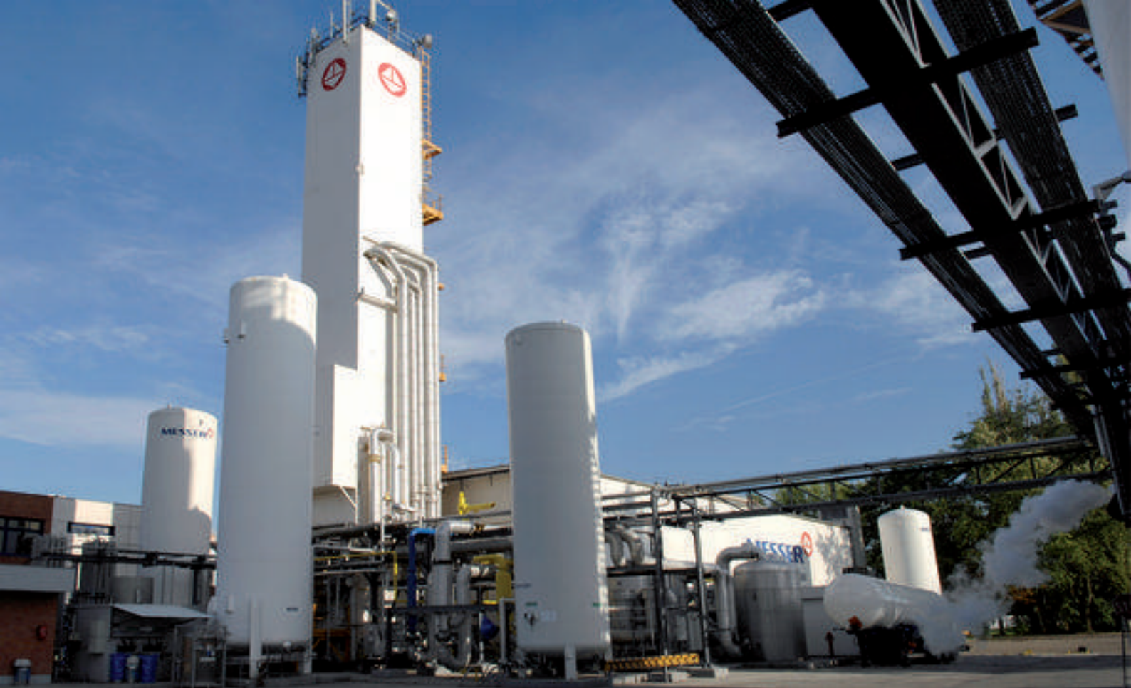
Air separation unit at Messer in Hungary
