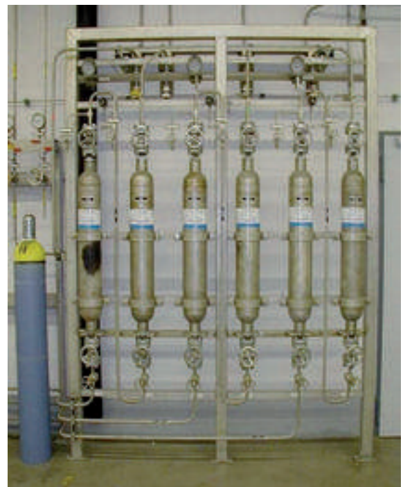
Figure 11: Oxisorb® purifying station
