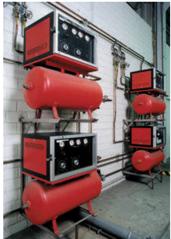
Figure 10: Nitrogen/hydrogen-mixer for gas mixtures
